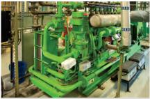
Captures methane from the treatment process to generate electricity and heat energy
