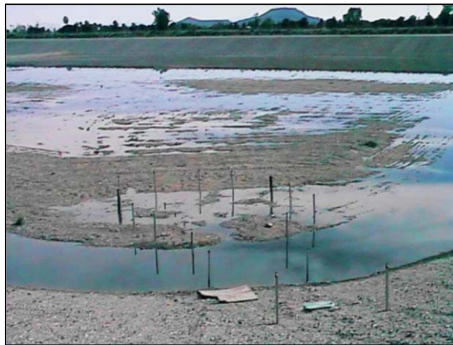
Figure 4-3 Recharge Basin Drying Cycle
