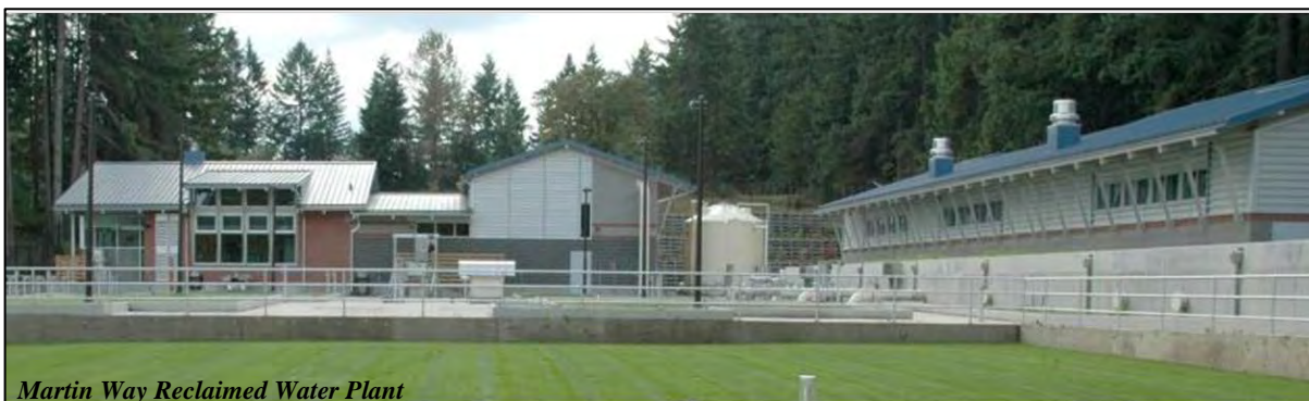
Martin Way Reclaimed Water Plant
