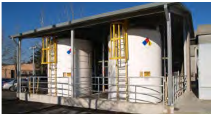
Direct Operating Expense accounts for all the non-personnel costs associated with the wastewater treatment process, such as operating supplies, utilities, chemicals, and tools.
