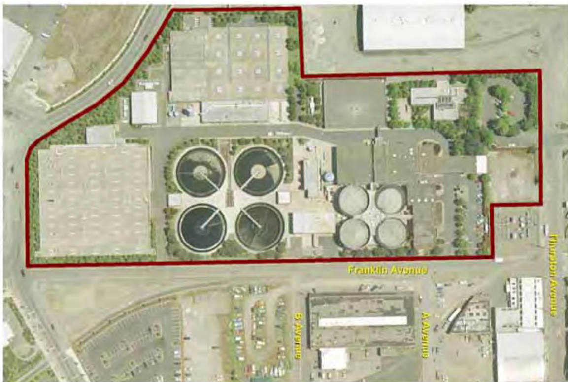
Figure 1-1. Budd Inlet Treatment Plant Site
