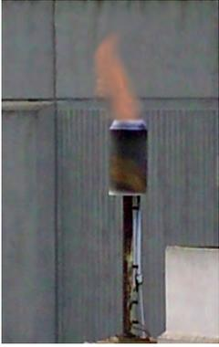
Excess methane-rich digester gas was previously handled through flaring. Flaring of the gas was wasteful, since this gas could otherwise be used to produce heat and/or energy. Additionally, an average of 14% of the methane had been escaping to the atmosphere. Methane is 21 times more damaging than carbon dioxide as a greenhouse gas.
